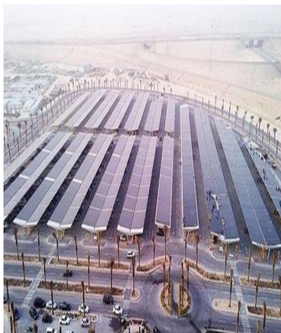
Fig. 2. The 10 MW Photovoltaic Carport System in Saudi Arabia [20].
